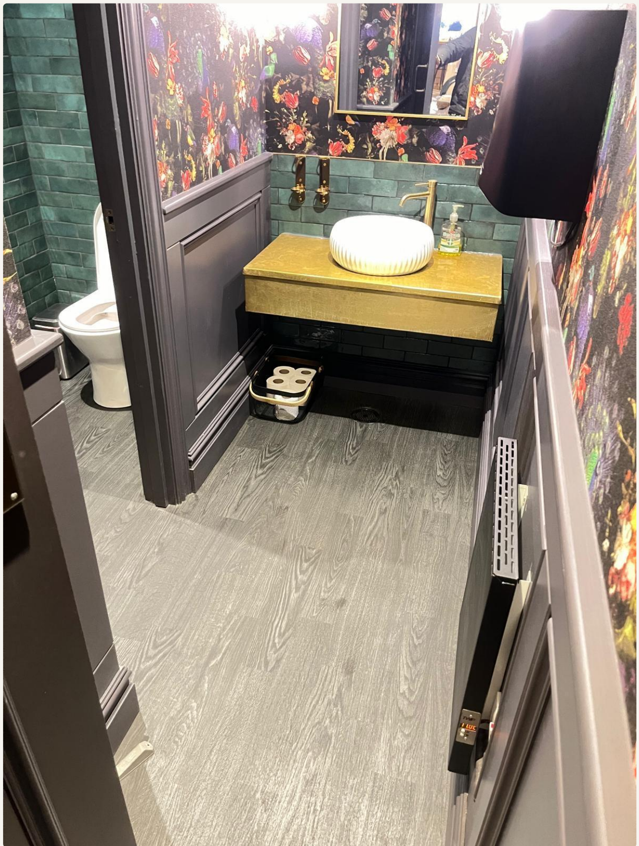
Finished ladies' washroom: the grey Amtico floor sits cleanly against the decorative wall covering and gold vanity unit, cut precisely to the room's angles.
